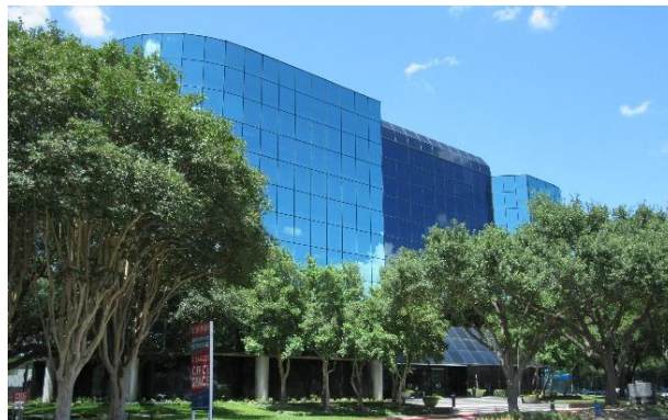
JBAH office is located on the 1 st floor of this 6-story building.
